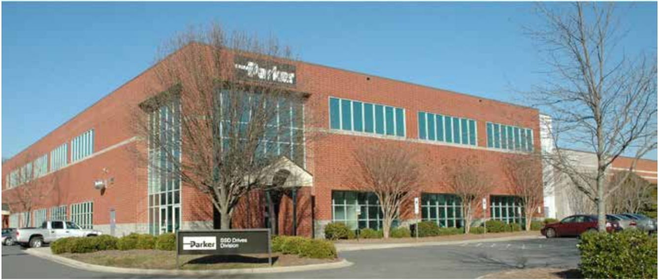
Parker Electromechanical & Drives Division Headquarters - Charlotte, NC
